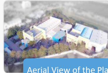
Aerial View of the Plant
